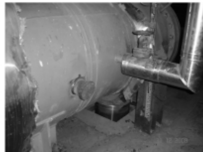
Figure 6: Holes made on the LPH shell were blanked.
